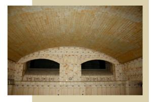
The regenerative end fired furnace is the type of furnace mainly used for container glass, table ware, pharmaceutical glass, sheet glass and sodium-silicate glass. It's melting range is typically from 30 – 500 TPD.
